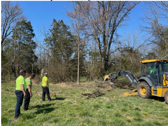
Public Works employees using a backhoe with a “thumb” to pull down netting, cables and to bring down telephone poles.
